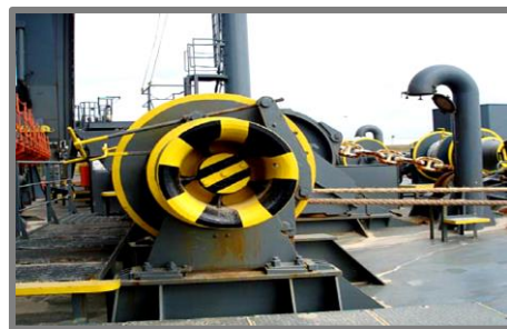
[Mooring station with effective hazard markings]
